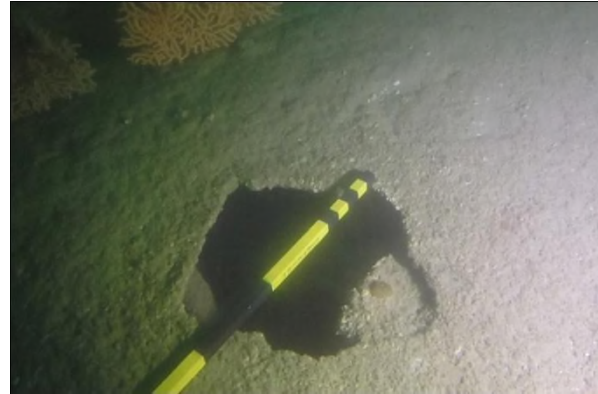
Figure 56: Hole H1 on the starboard side
